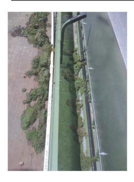
This picture illustrates why grass clippings easily clog pumps and lines. Notice how dry the waste material is light and easy to land fill.
